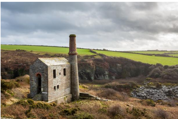
Verlassenes Cornish Engine House
